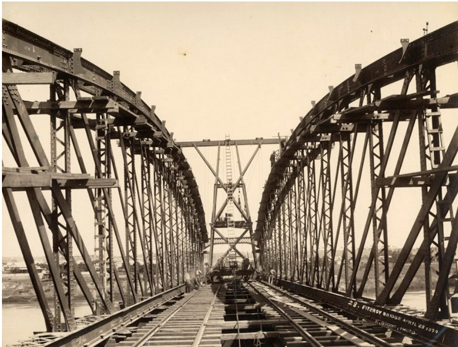
Construction of the Alexandra Bridge, Rockhampton, Henry Goode. Courtesy Queensland Museum Network Collection
