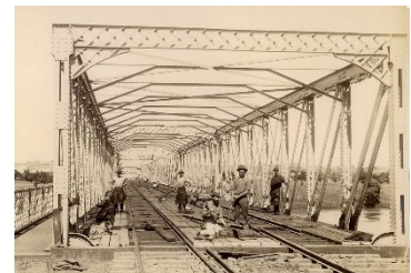
Construction of the Alexandra Bridge, Rockhampton © Queensland Museum
